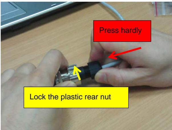
Step 9: Tighten the plastic rear nut again to make sure the cable is securely connected and would not fall off accidentally
