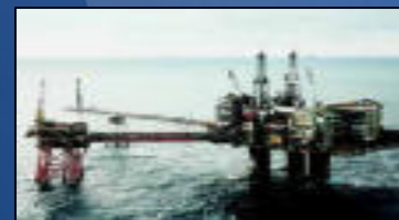
REMOTE PROCESS MONITORING
